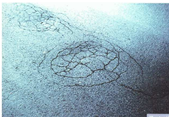
FIGURE 2.6. Faïençage circulaire [LCPC, 1998]
